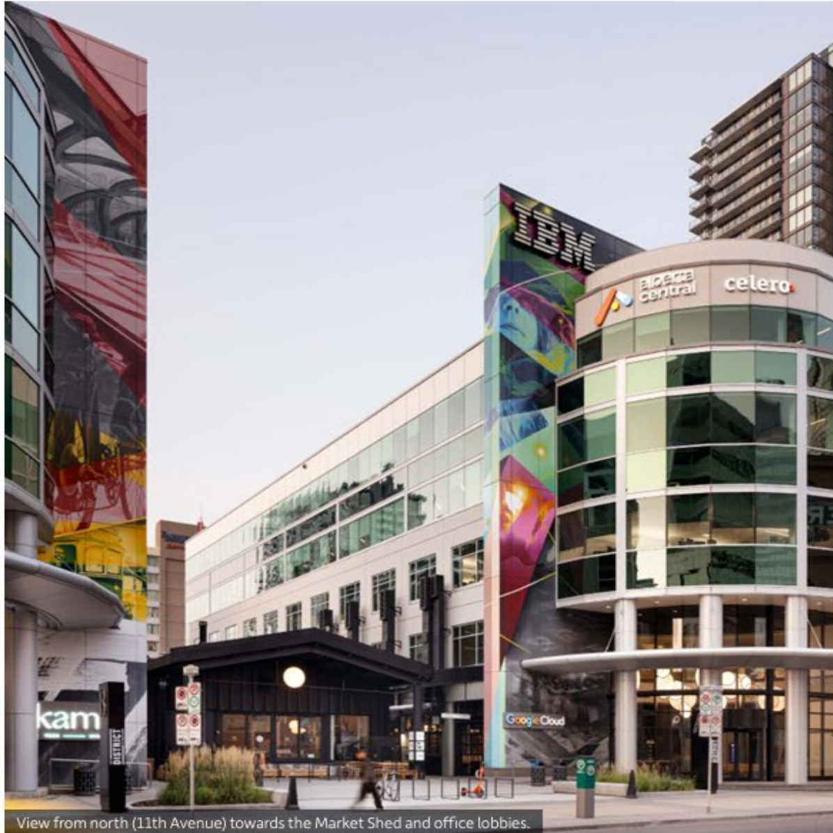
View from north (11th Avenue) towards the Market Shed and office lobbies.
